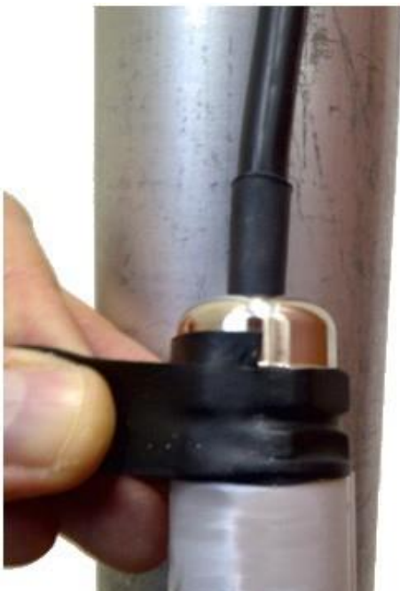
Figure 2-67: Waterproofing an external connection
