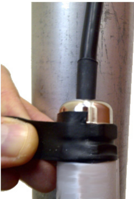
Figure 2-67: Waterproofing an external connection
