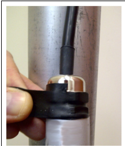
Figure 2-25: Applying sealant tape to an external connection
