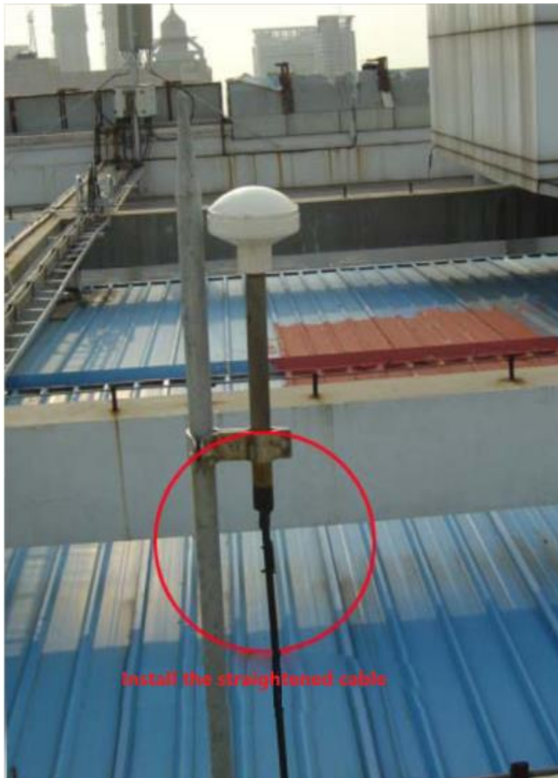
Figure 3-30 No cable allowance
