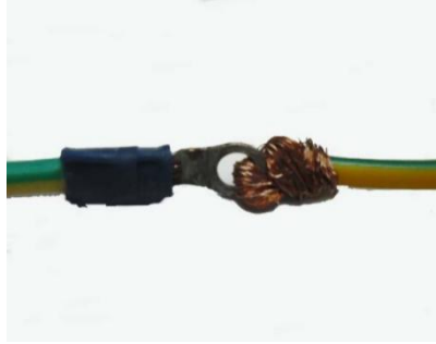
Figure 3-14 Grounding wire connection
