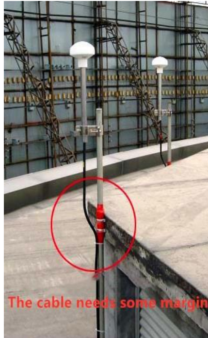
Figure 3-22 Installation diagram of antenna feeder
