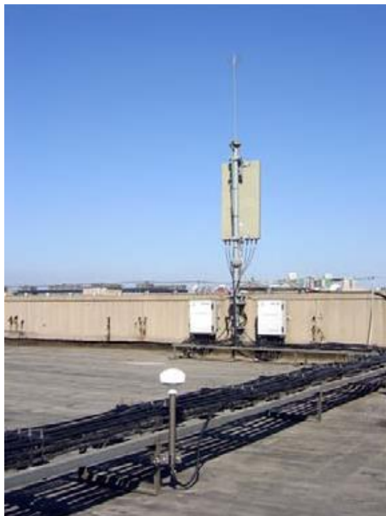
Figure 3-28 The antenna is too close to the cable rack
