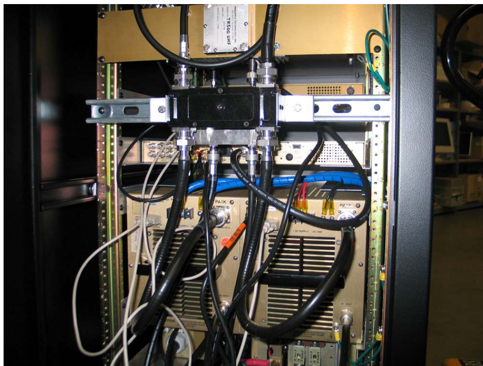
Rear Door Open Middle Third View
