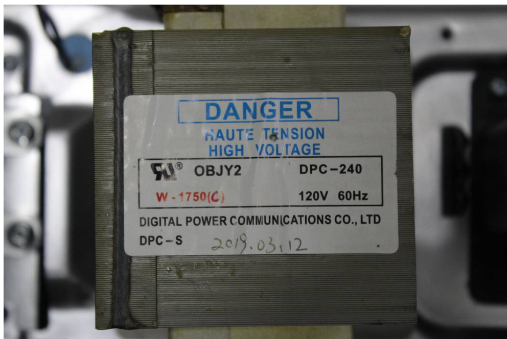
EUT –Transformer View
