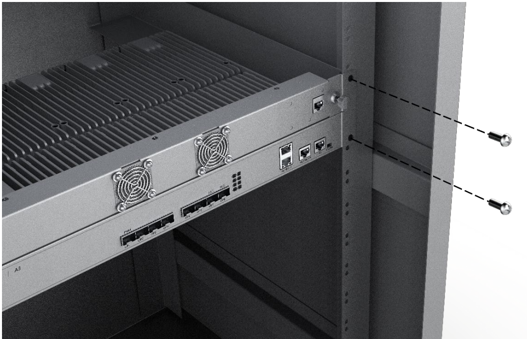
Figure 5. Place A3 in Rack
