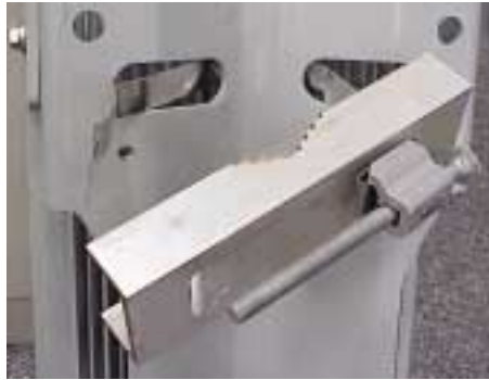
figure 56. banding through cSPICE bracket
