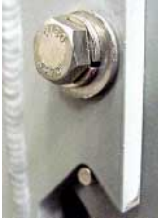
figure 30. bolts and washers (top) and hanging studs (bottom)
