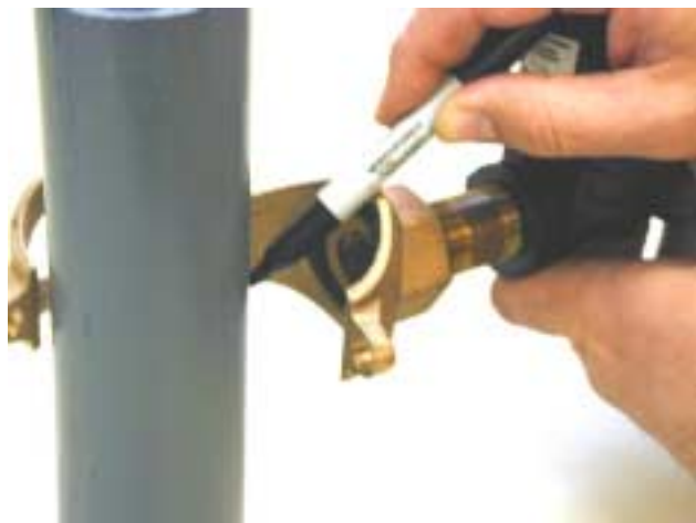
Figure 2-6. Marking Pipe
