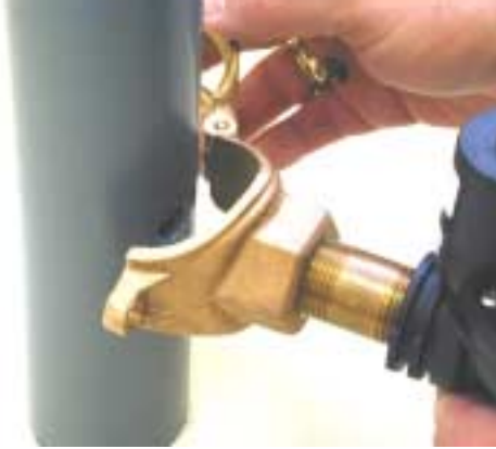
Figure 2-9. Attaching Solenoid Valve Assembly
