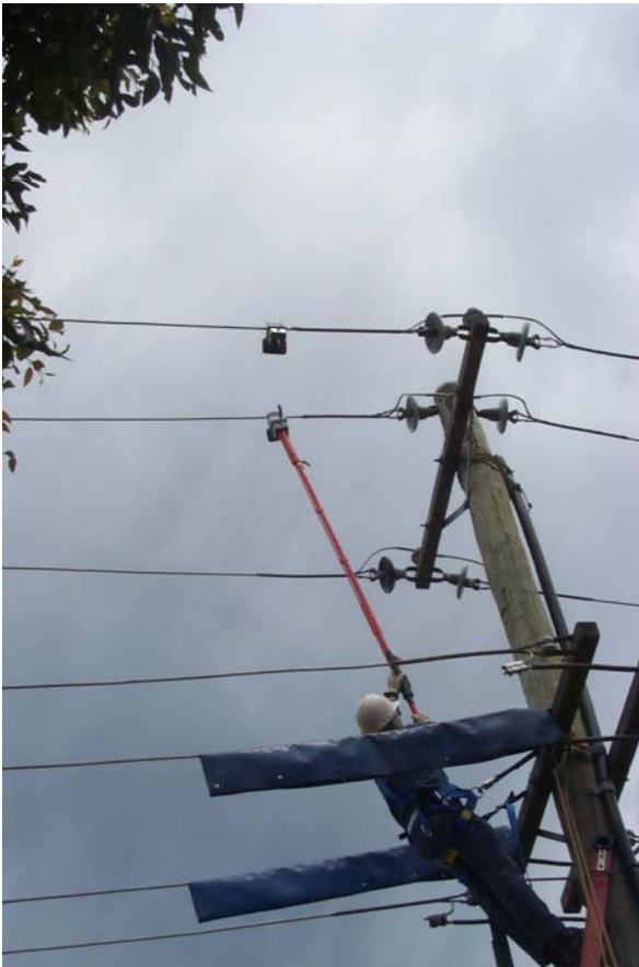
Figure 2: LT40 CMS Installation via Hotstick
