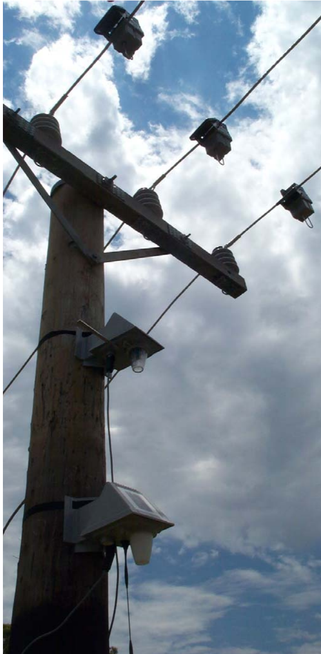
Figure 6: Example Installation showing LT40CMS, LT40PAC and cellular modem.
