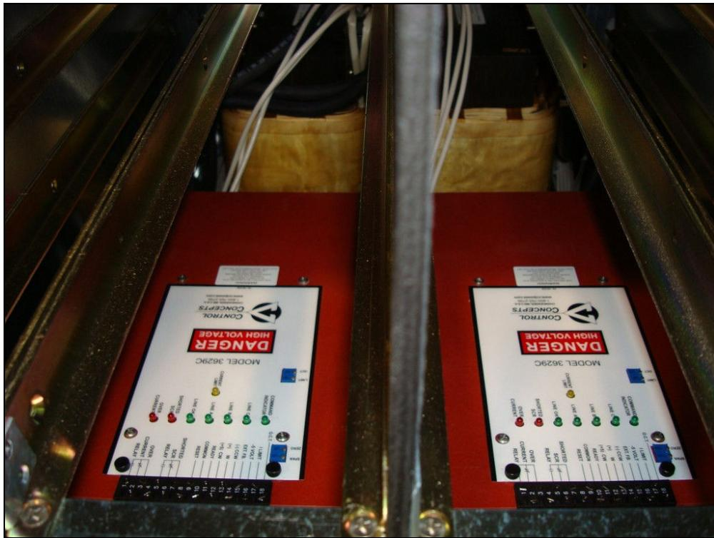
**6.13 Front view – Load Regulator Assembly (RF Amplifier Cabinet)**
