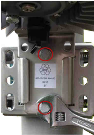
Figure 14: iR460 Installed on a Large Pole
