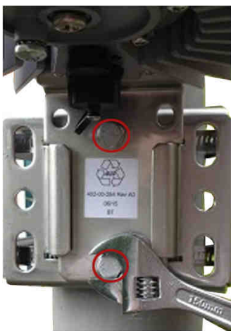
Figure 9: Securing the iR460 Unit
