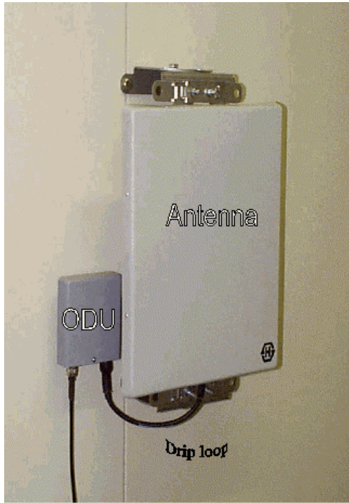
Figure 3-1 High Gain Panel Antenna Installation
