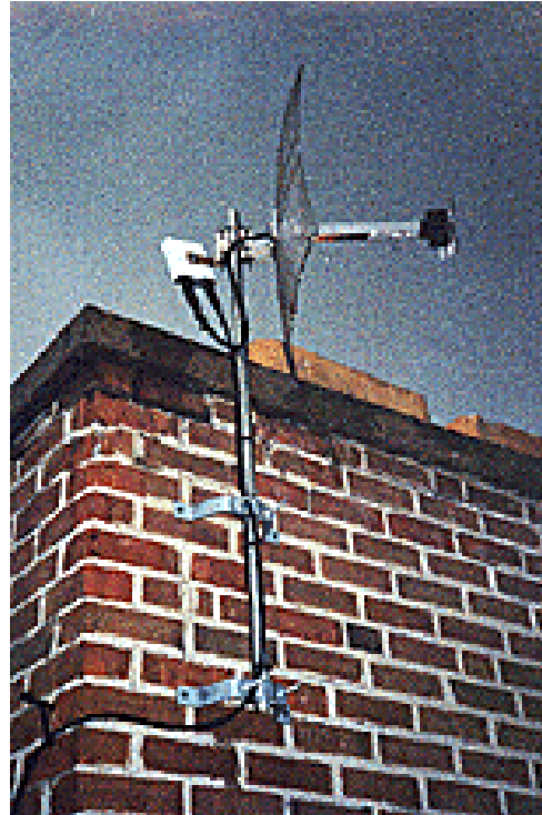
Figure 3-2 High Gain Reflector Antenna Installation
