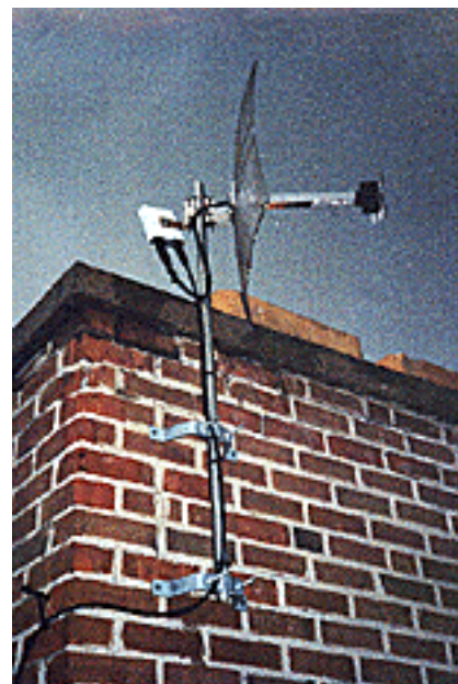
Figure 3-3. High Gain Reflector Antenna Installation
