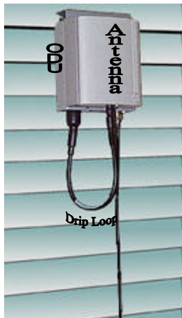
Figure 1-8. 9714-2820 Low Gain Panel Antenna Assembly
