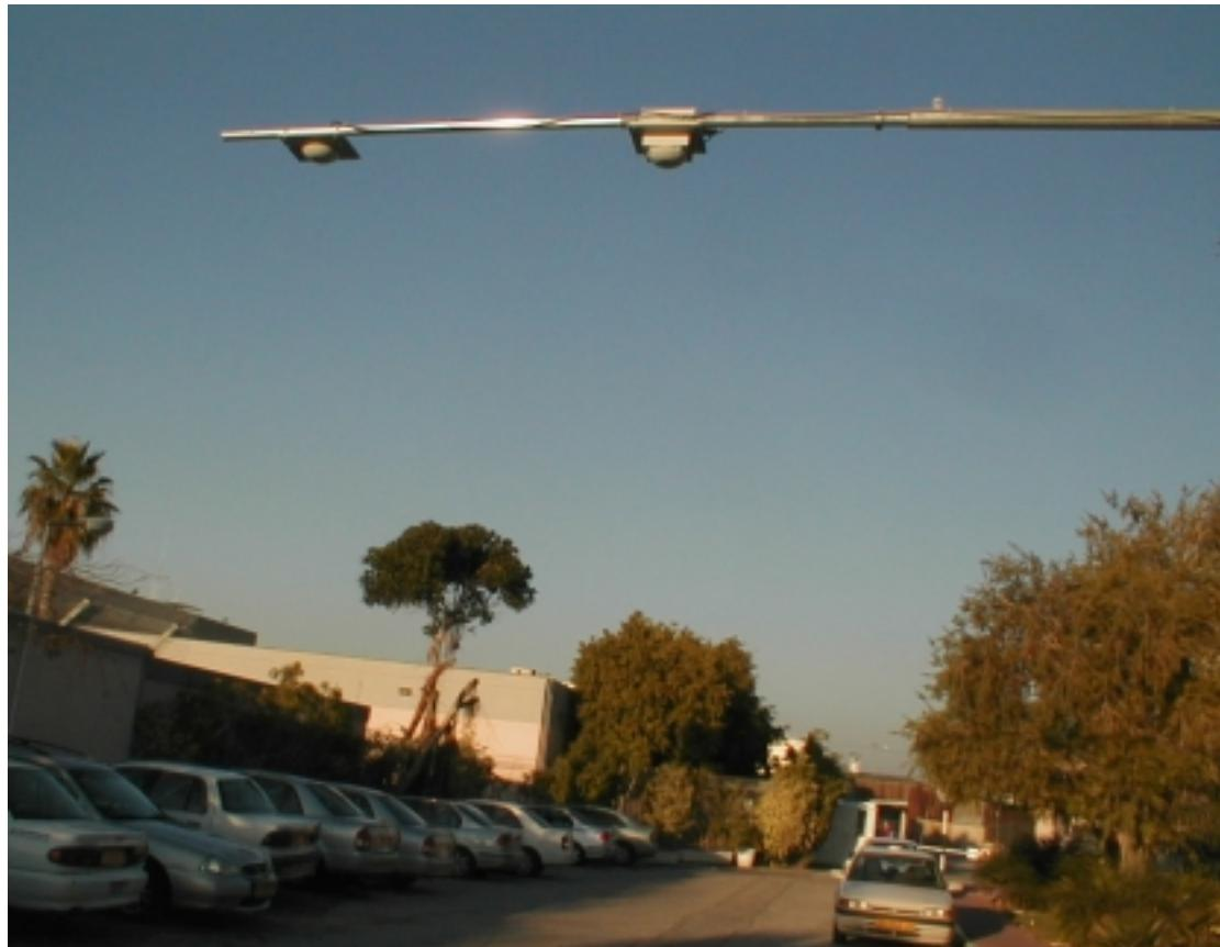
The pipe has to be 1.5" up to 2" in diameter, and its length has to be sufficient to locate the RSC over the center of the lane. (The width of a standard lane is about 3.6m  $\cong$  12ft). For longer pipes and for areas with extreme winds it is important to add additional supports (stilts, cables, etc.) to prevent bending of the pipe.
