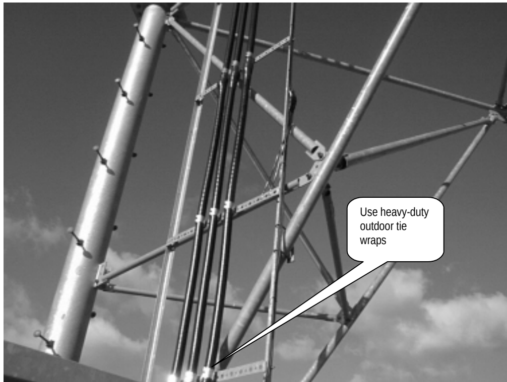
Figure 2-3. Fasten IF Cables to the Tower
