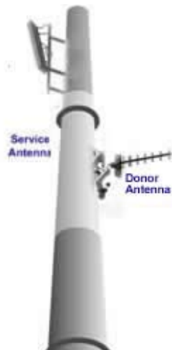
Figure 2-1. Service above Donor Antenna
