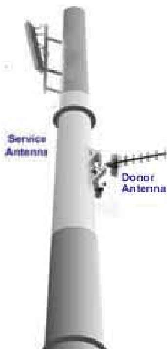
Figure 2-1. Service above Donor Antenna
