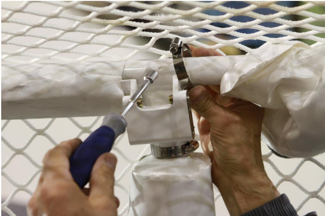
Installing Pipe-clamps to Bracket
