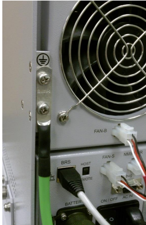
Figure 22 Ground Cable Connection
