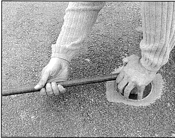
STEP 26 - Secure lid by tightening with lid tool.
