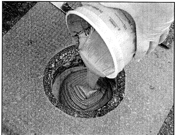
STEP 13 - Immediately pour the epoxy mixture into the hole.
