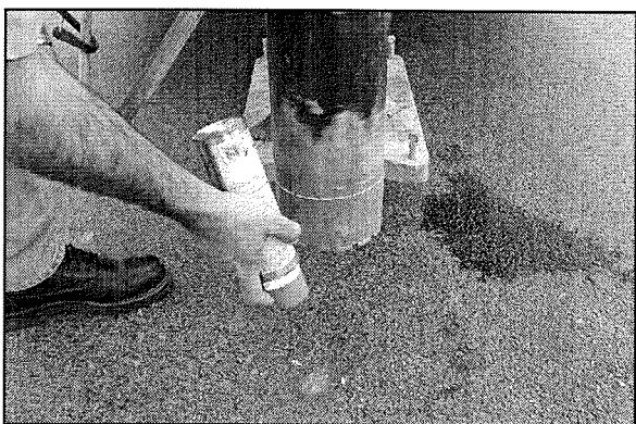
**STEP 1** - Locate the center of the traffic lane and mark the road with paint. This will be the location (center of lane marking) of the Groundhog canister.
