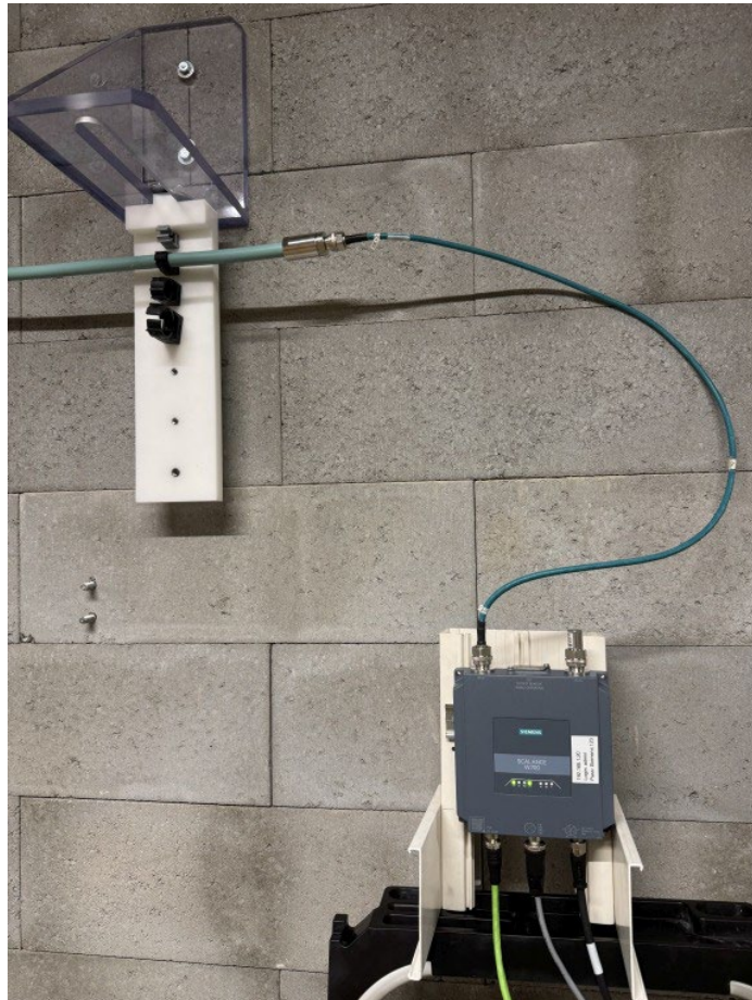
Photo 1: Installation of EUT with connection to RCoax cable
