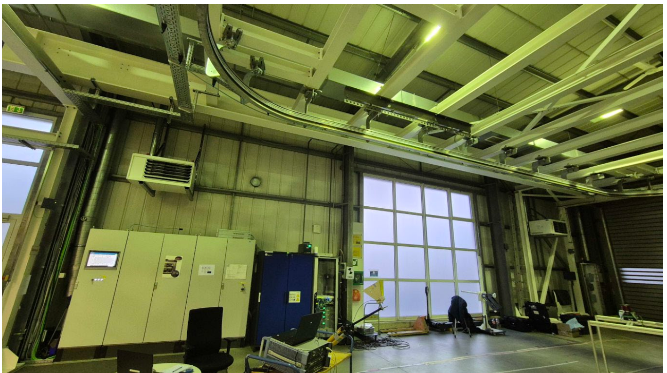
Photo 4: Test location overview
