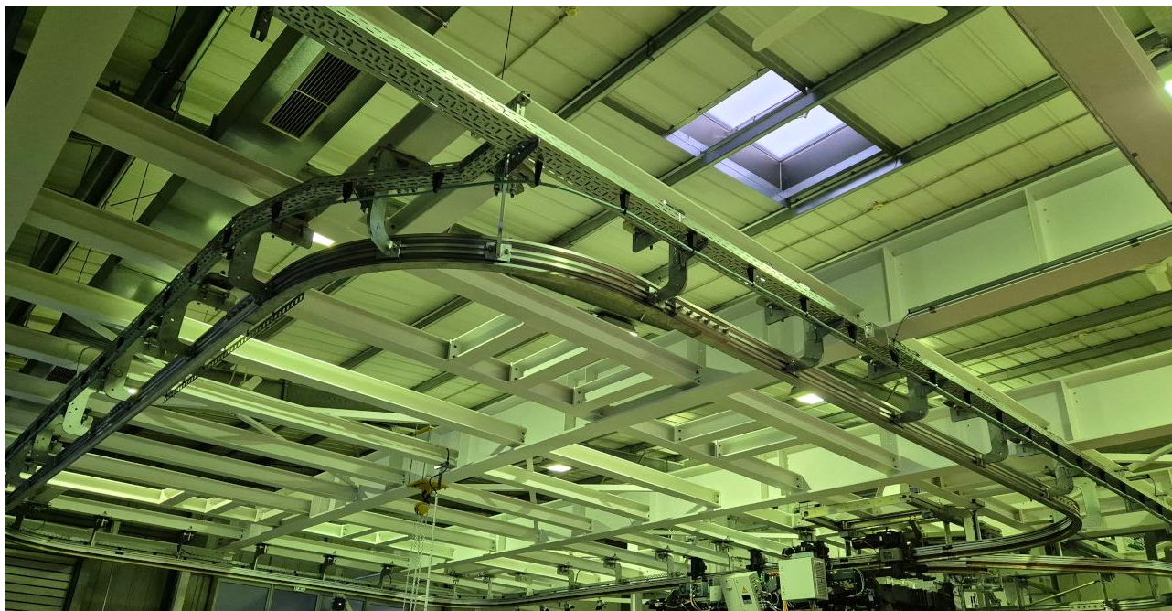
Photo 2: Installation of RCoax cable in the test location
