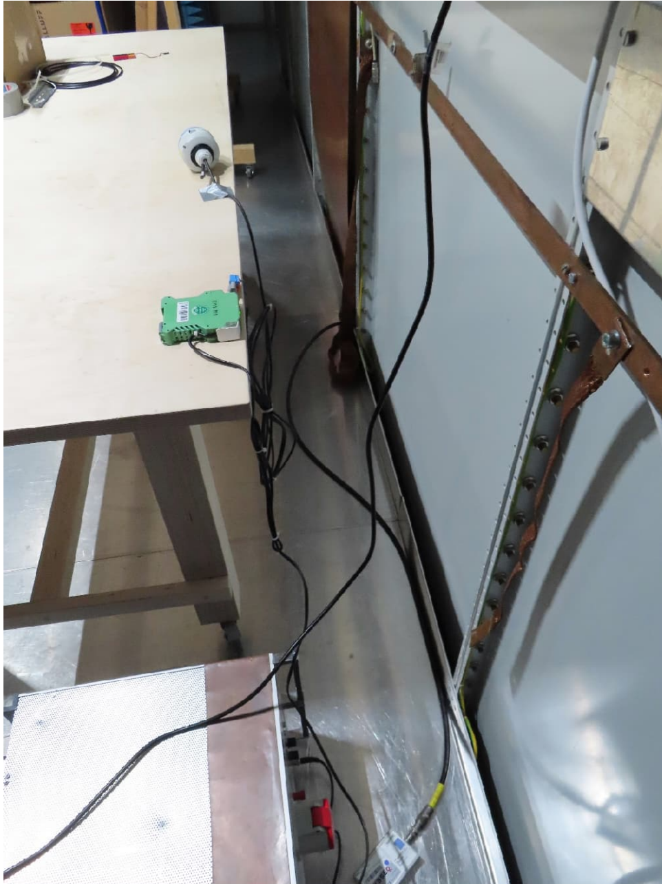
Test setup – power-line conducted
