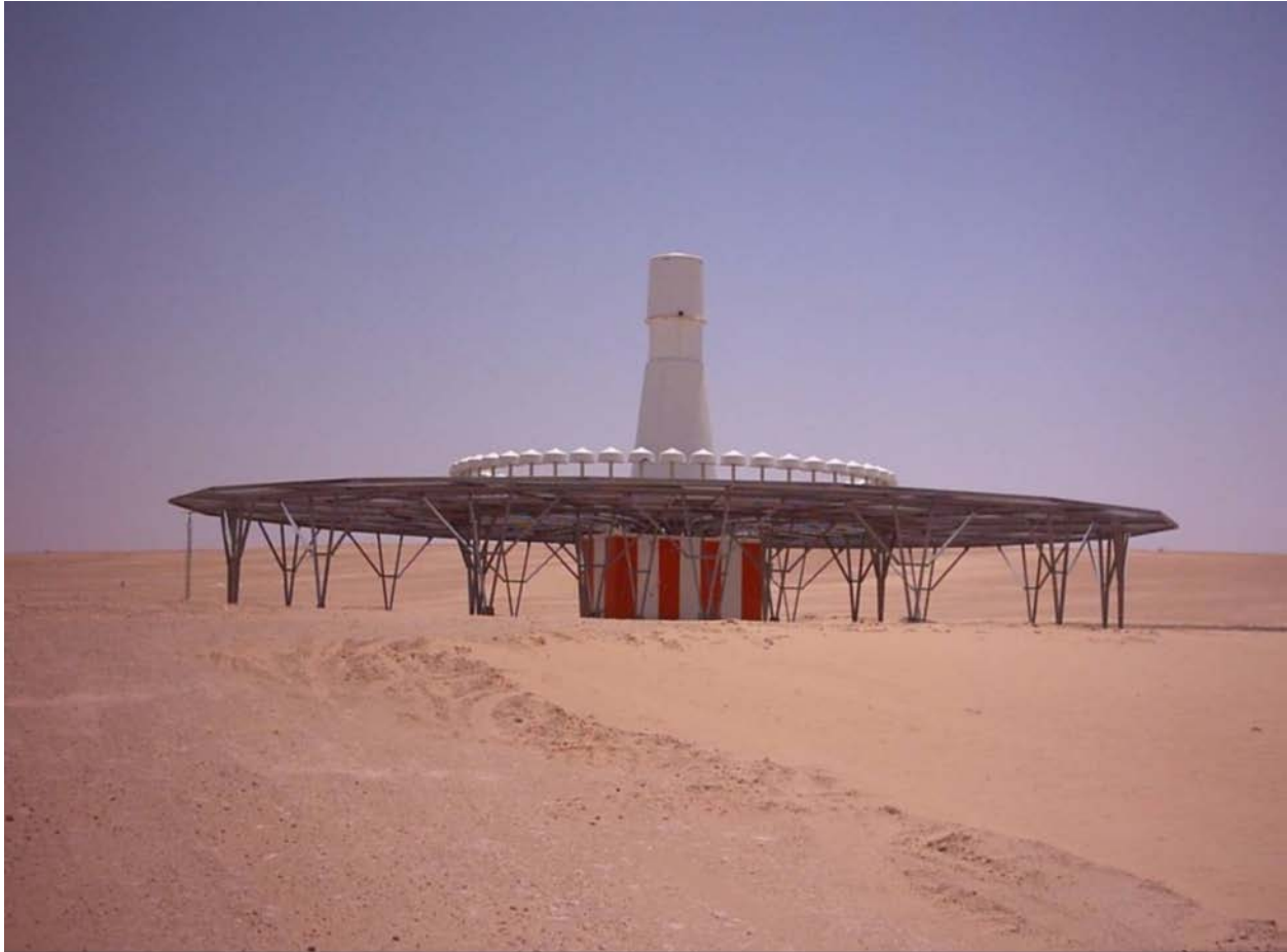
Figure 1-1 Dual Doppler VHF Omni-range (DVOR) Station with TACAN
