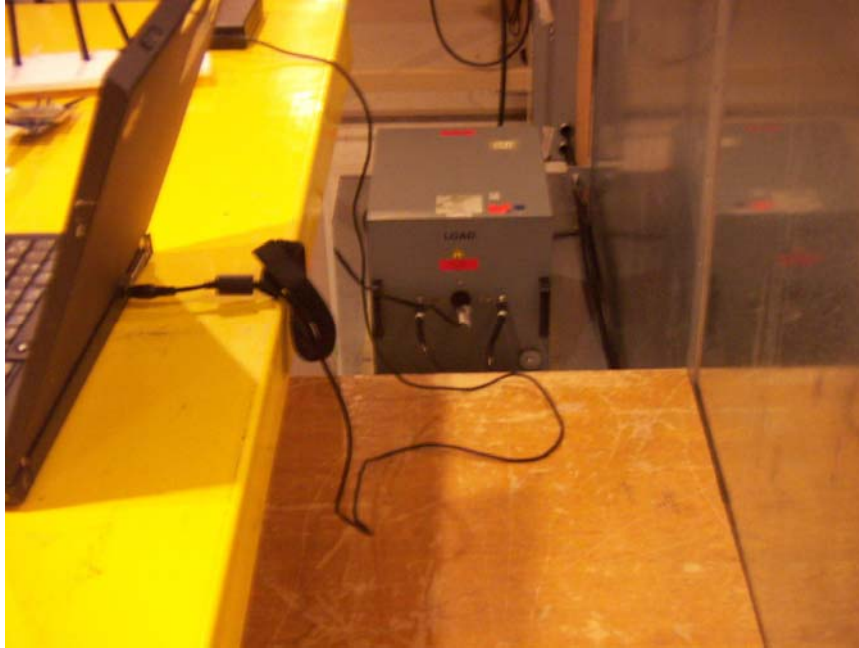
LINE CONDUCTED BACK PHOTO
