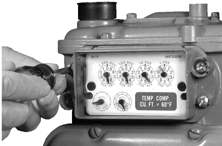
Figure 3: Cover Removal
