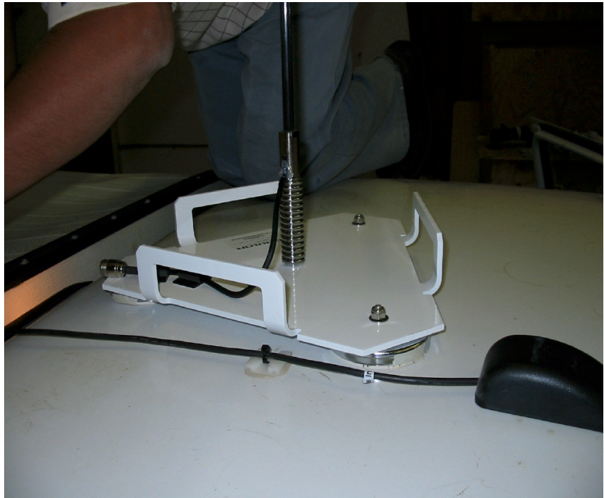
Figure 2.14 RF Antenna Location
