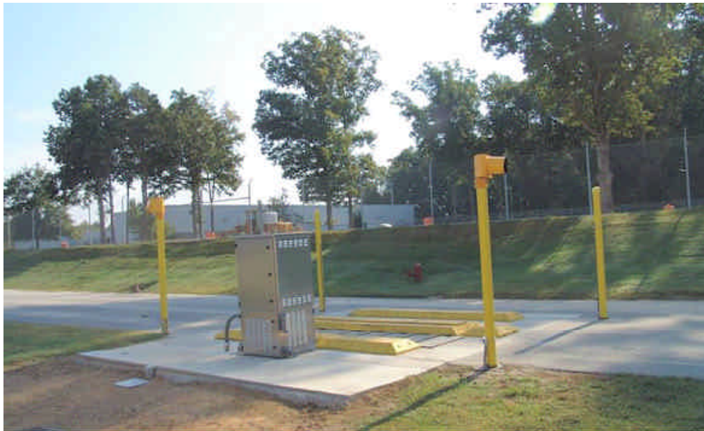
Fig 1: The Drive-By-Reader (DBR), including control unit and antenna array.
