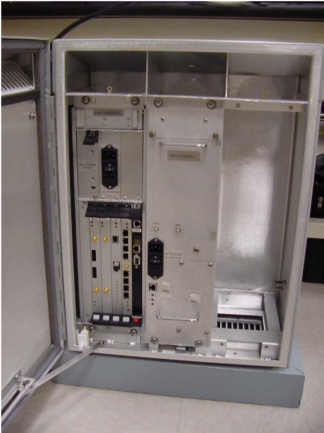
RAN Disassembly - Open View
