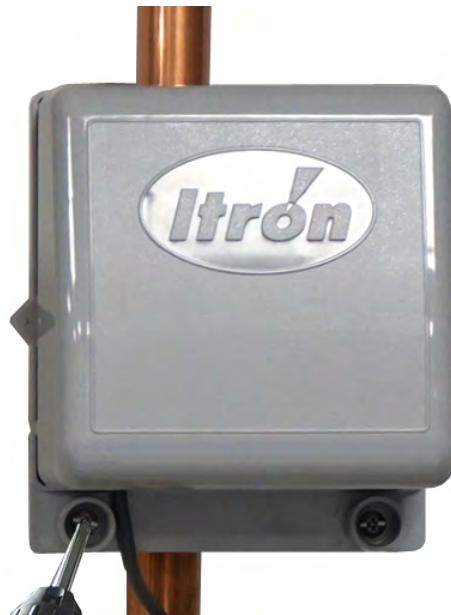
4. Tighten the screws to 9 to 12 inch-pounds of torque.
