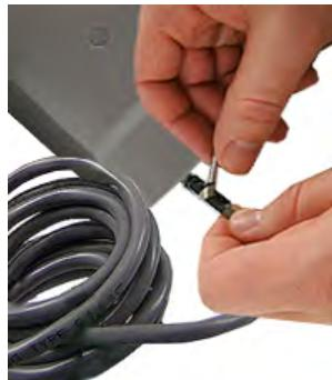
4. Beginning over the installed electrical tape, twist the Itron cable armor onto the remote 500W ERT module cable using a right-handed twist.
