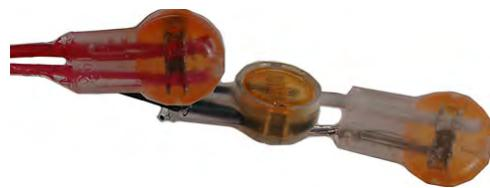
6. Insert the connectors and wires into the splice tube until the connectors and wires are completely immersed in the non-conductive gel material.
