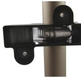
5. Tighten the clamp screw three or four more turns to make sure the end of the band does not pop back out on this side of the pipe bracket. Verify the pipe clamp is in the final installation position on the pipe and completely tighten the band clamp screw.
