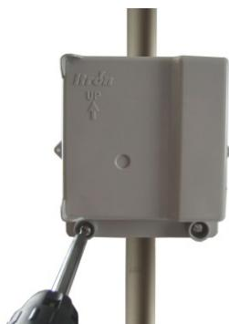
4. Tighten the screws to 9 to 12 inch-pounds of torque.
