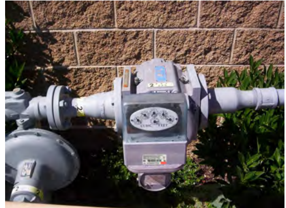
Sensus commercial ERT Module mounted on a Dresser meter with an instrument drive
