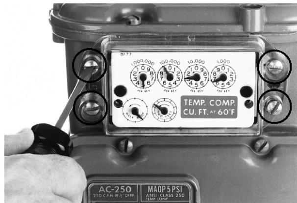
3. Examine the index cover screws you removed. Verify they are 5/8-inch long and not corroded.
