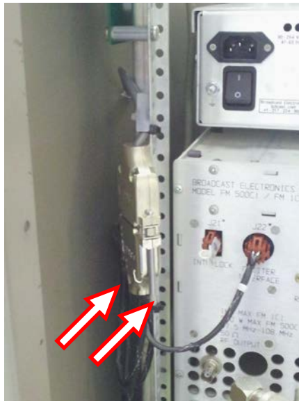
Figure 13 – Exciter Interface Cable
