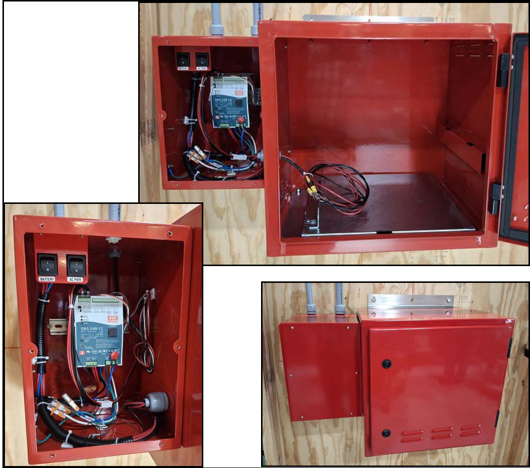
Figure 4-7 CS19-BBU-005 battery cabinet without battery installed
