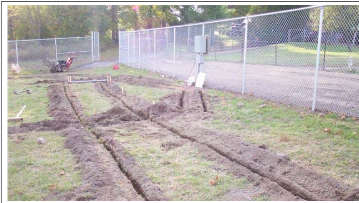
Trenches for lead-in cables to the Microtrack Processor.
