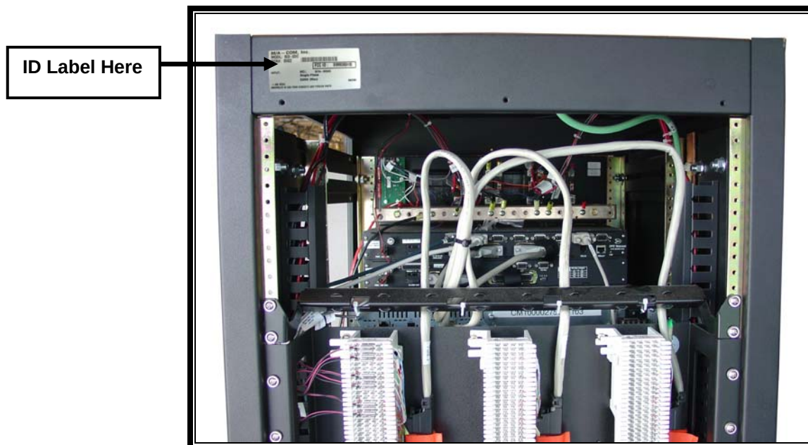
Photograph 2: ID Label Location
