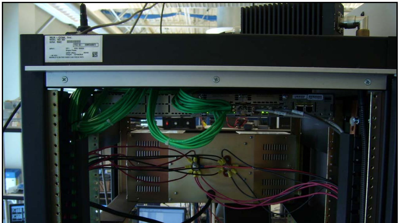
Photograph 2: ID Label Location
