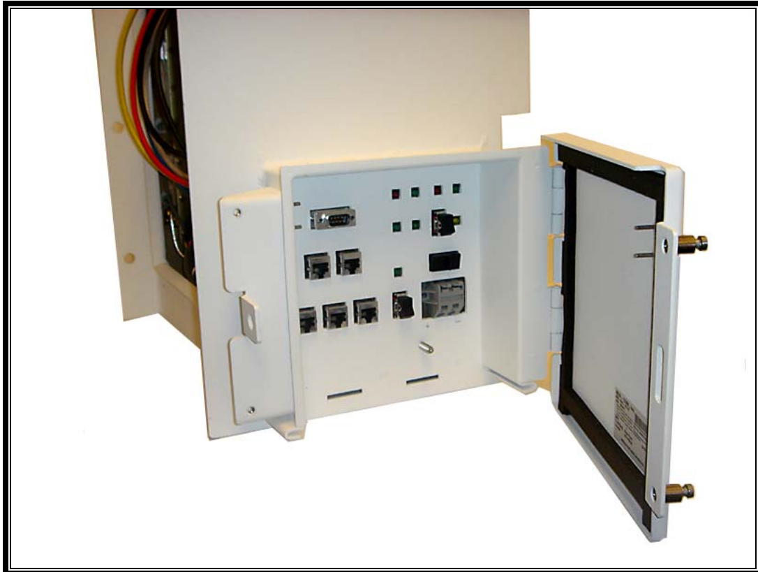
Photograph 5: 900 MHz Cell Site – Front View
