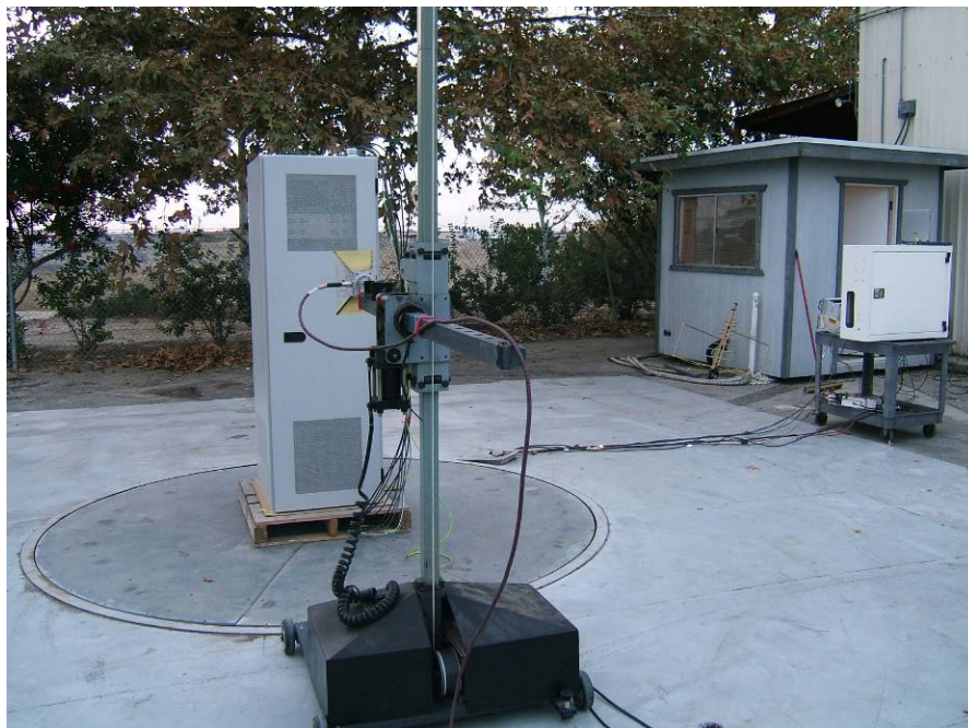
Glideslope Test Setup Photo
