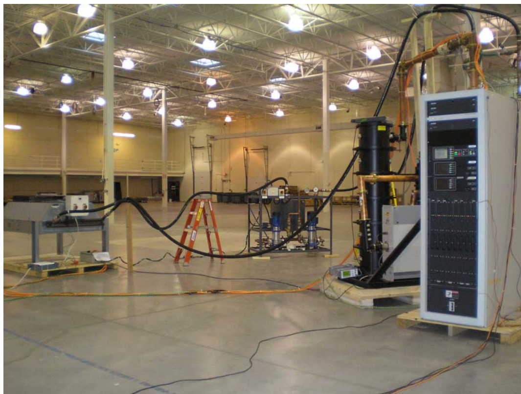
Transmitter and ancillary equipment (Pump Module and Heat Exchanger)
