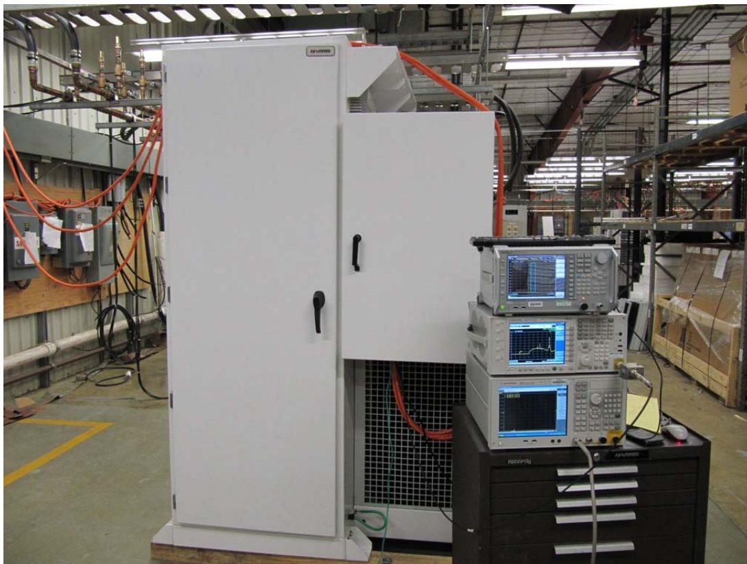
Figure 9, Spurious Test Setup
