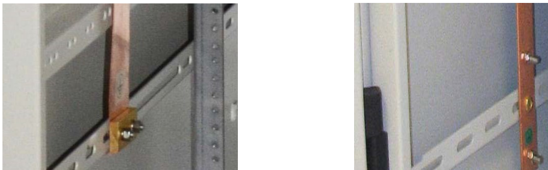
Figure 2-2 Cabinet Ground Buss Bar Connections
