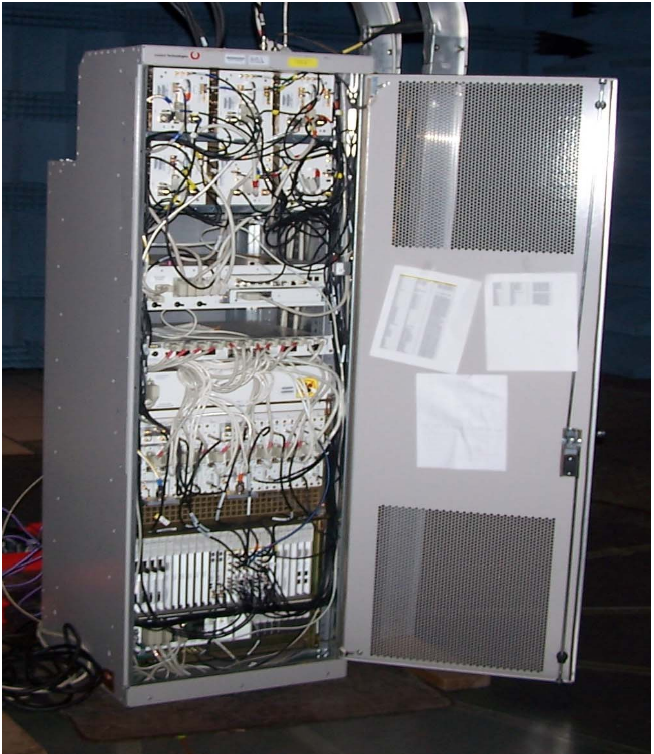
AS5ONEBTS-24 Alcatel-Lucent t Base Transceiver Station (BTS) Front View – Door Open
