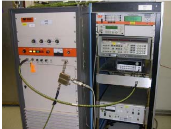
Support Equipment Setup
