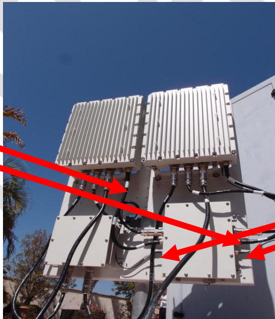
Figure 11: Cable installation between units
